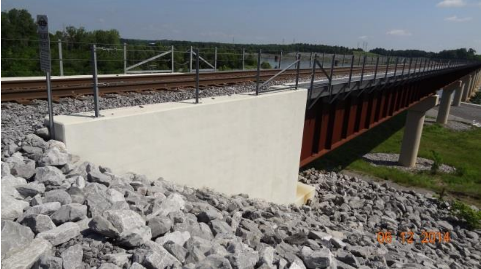
FIGURE 4 West End of Site #1 Bridge Transition Zone.
