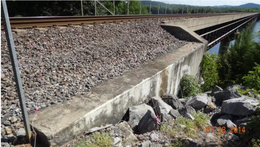
FIGURE 7 West End of Site #2 Bridge Transition Zone.
