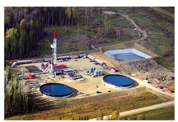
FIGURE 1 Well pad liner installation around drill rig and other containment areas.
