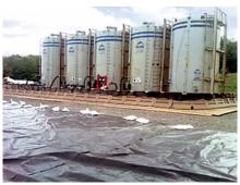
FIGURE 3 Secondary containment for steel oil and gas storage tanks.
