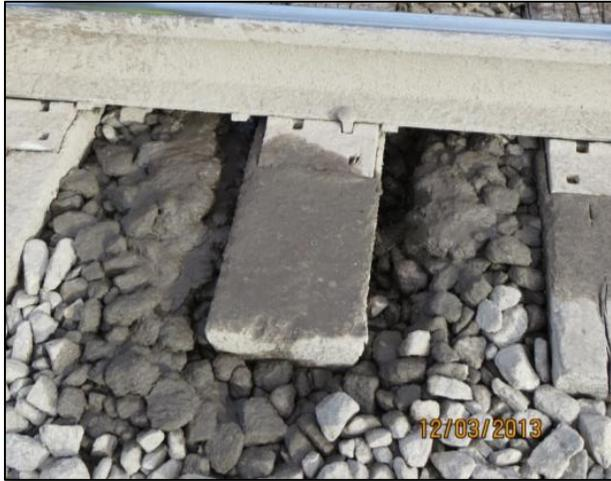
**FIGURE 6 – PHOTOGRAPH OF WET, FOULED BALLAST**
