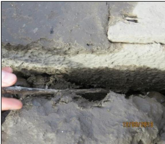
**FIGURE 7 – PHOTOGRAPH OF A GAP UNDERNEATH A TIE IN WET, FOULED BALLAST SECTION OF TRACK**
