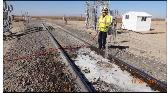
**FIGURE 8 – PHOTOGRAPH OF THE FULL SOAKING OF A SECTION OF FOULED BALLAST TRACK**
