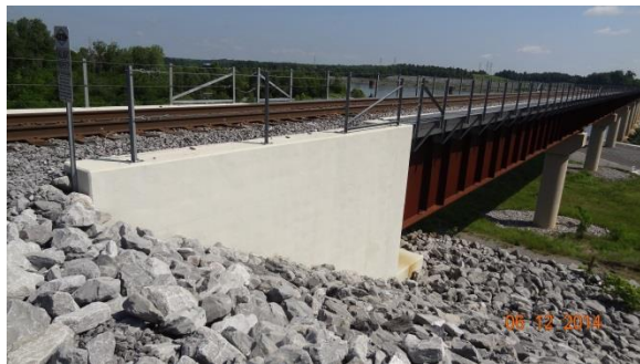
FIGURE 1 – WEST END OF SITE 1 BRIDGE TRANSITION ZONE
