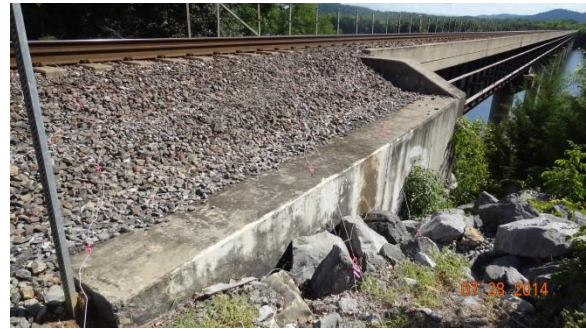
FIGURE 2 – WEST END OF SITE 2 BRIDGE TRANSITION ZONE
