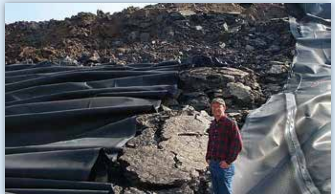
Figure 3. Failed slope and damaged geomembrane.
