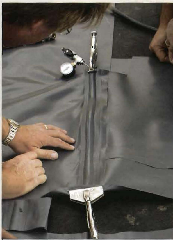
Photo 3. Air-channel testing of T seam in 30 mil sheet.
