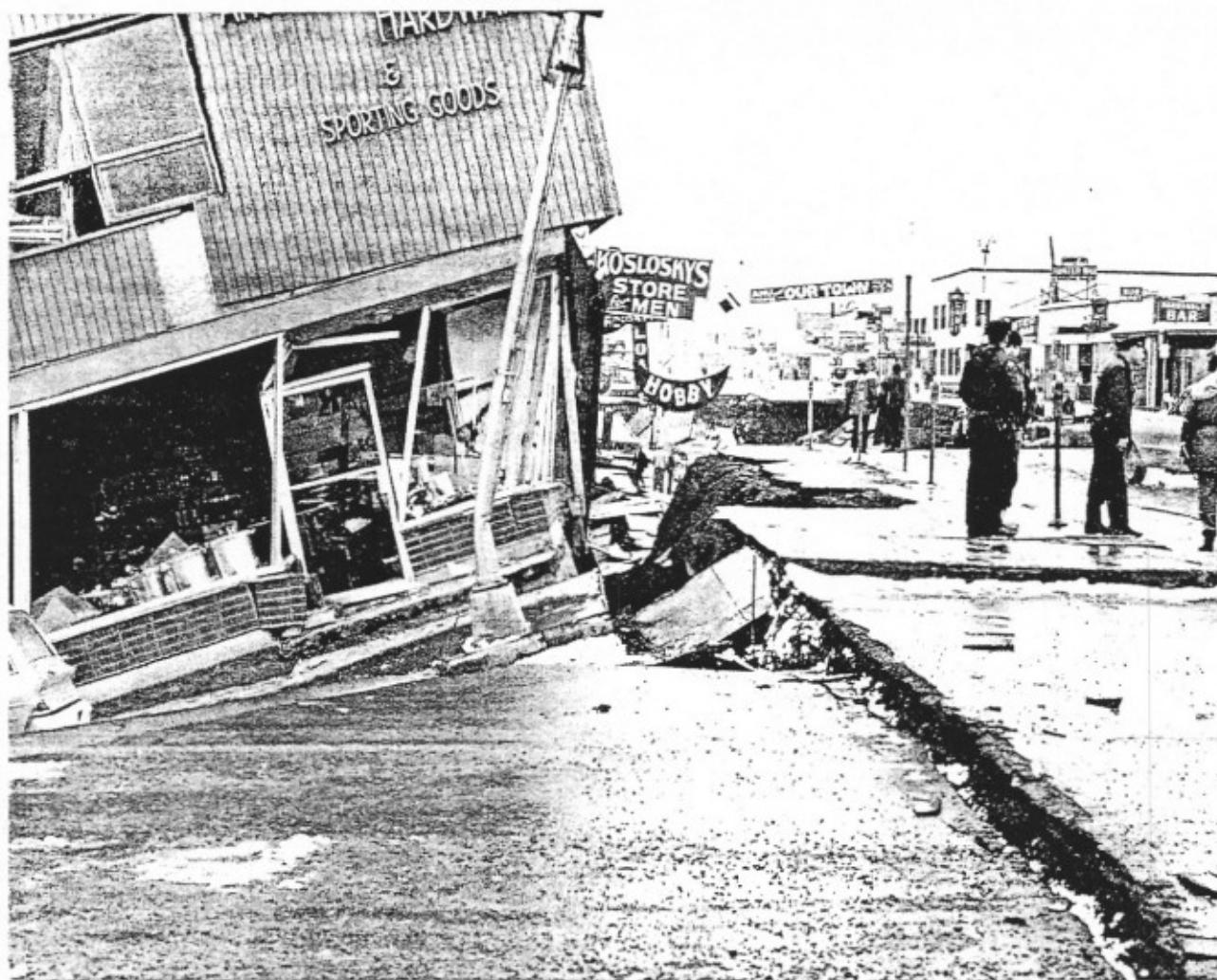
FIG. 1. View of Damage and Scarp in Fourth Avenue Landslide
