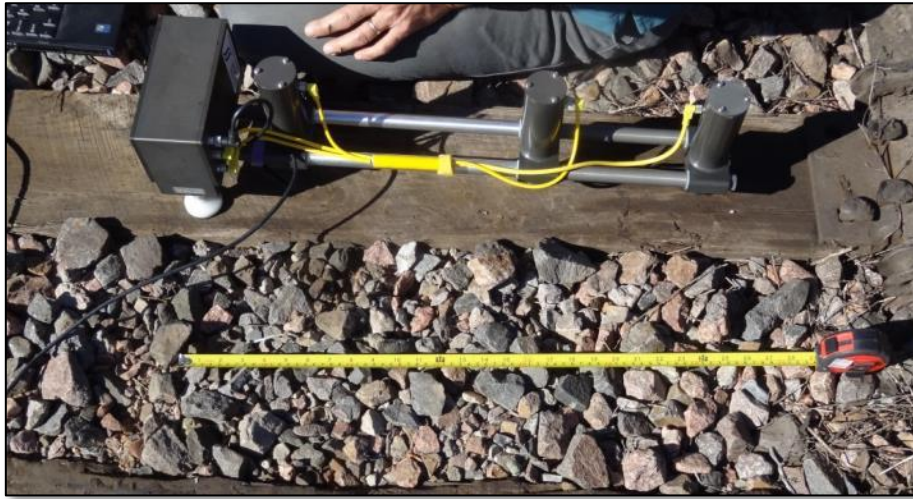
Figure 3. Photograph of the BSPA system measuring the modulus of a timber tie
