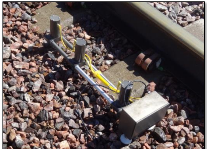
Figure 2: Photograph of BSPA measuring ballast modulus under a concrete tie
