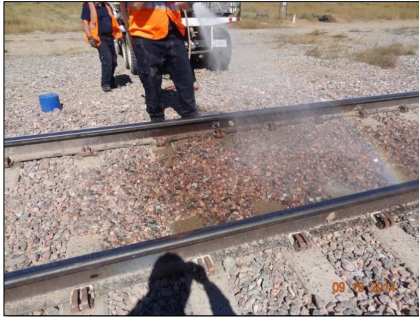
Figure 5: Photograph of wetting of a section of clean ballast track
