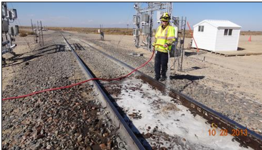
Figure 8: Photograph of the full soaking of a section of fouled ballast track
