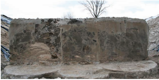
[FIG. 14] Cross-Section of Three JG columns in DTP Showing Significant Soil Inclusions.
