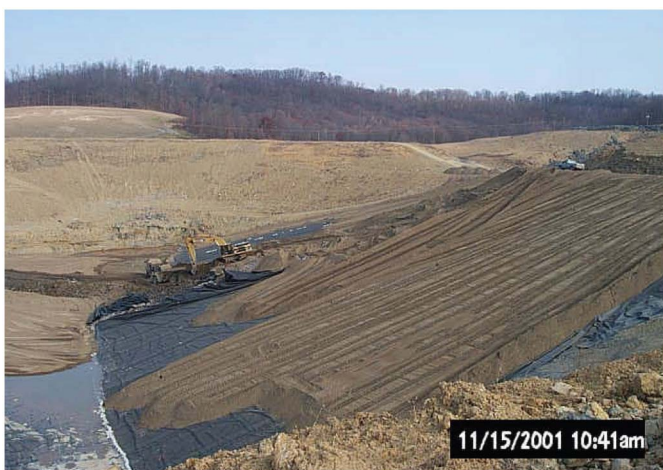
Fig. 2. Overview of sideslope and protective sand placement on geomembrane
