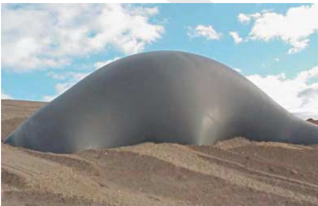
Figure 3. Inflation of PVC geomembrane by methane gas in landfill cover
