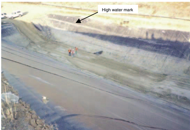
Figure 3. Sump area after pumping out storm water
