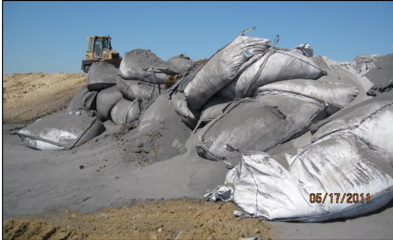
372 Figure 5: Sacks of baghouse dust being placed in APW monofill
