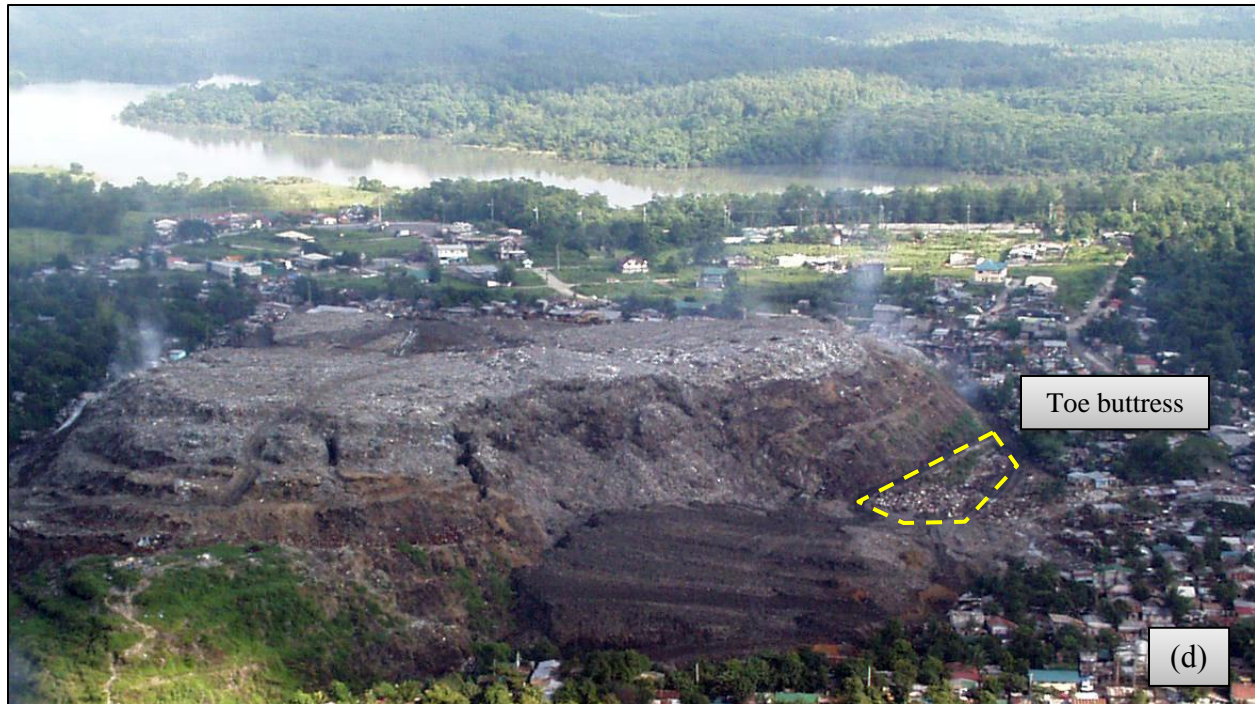
Figure 6. Slope geometry and failure surface after failure (photos by S.M. Merry).
