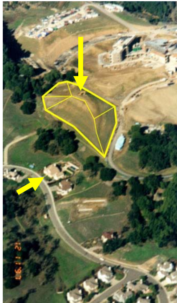
Fig. 5. Aerial illustrating size of landscape screen in relation to a 375 m 2 single family residence (see arrow) and an excavator on the top of the landscape screen (see arrow)
