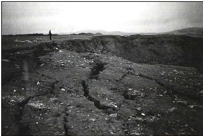
Fig. 4. Tension cracks on top of landfill and steep backscarp in MSW after slope failure (Kocasoy and Curi 1995)
