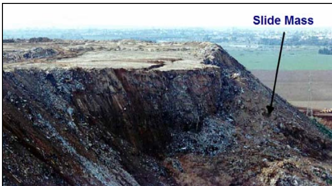
Fig. 6. 1997 Hiriya landfill slope failure (Isenberg, 2003)
