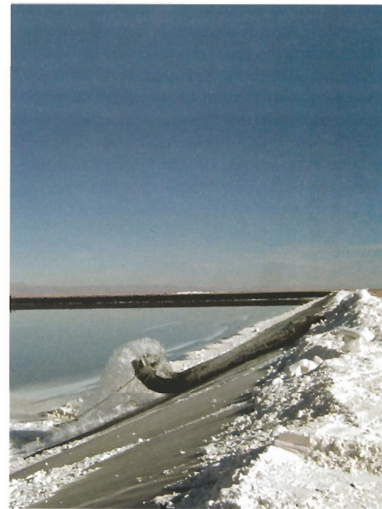
Photo 5 | A 3.28-million-ft. 2 (1-million-m 2 ) pond lined with PVC geomembrane filling with brine.
