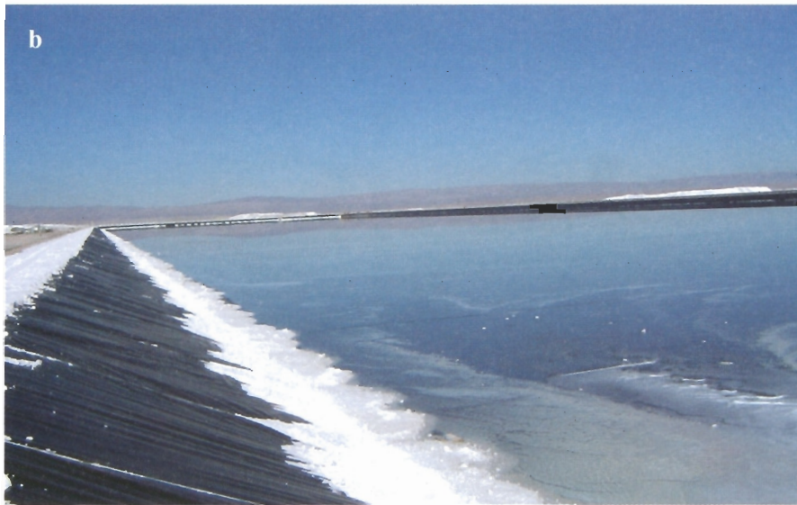
Photos 4a, 4b, 4c | A new evaporation pond, with the final liner installation completed (a), the pond in preparation for the brine (b), and brine filling the pond (c).
