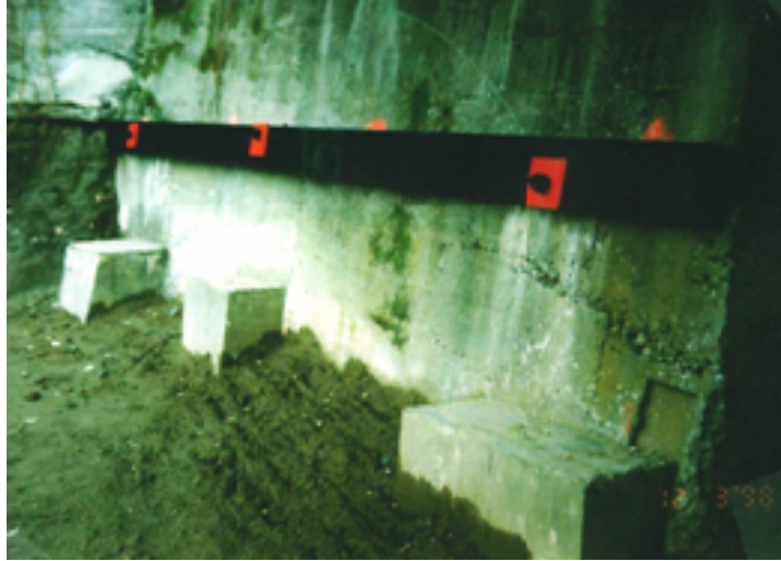
Figure 2: View of the anchors, waler beam, and encapsulated pier heads.
