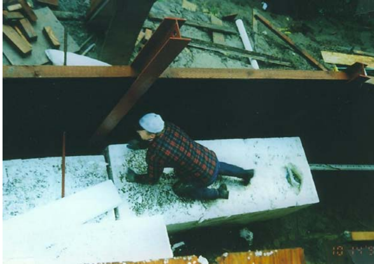
Figure 4. Geofabric block field installation
