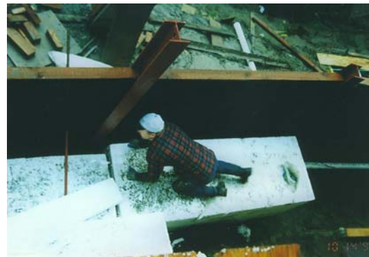
Figure 3. Geofoam block field installation.
