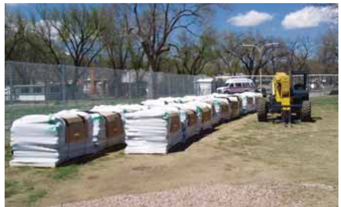
Photos 2 & 3 | Subsurface conditions included soft, high-plasticity clay. Sealed panels were shipped to the project site.
