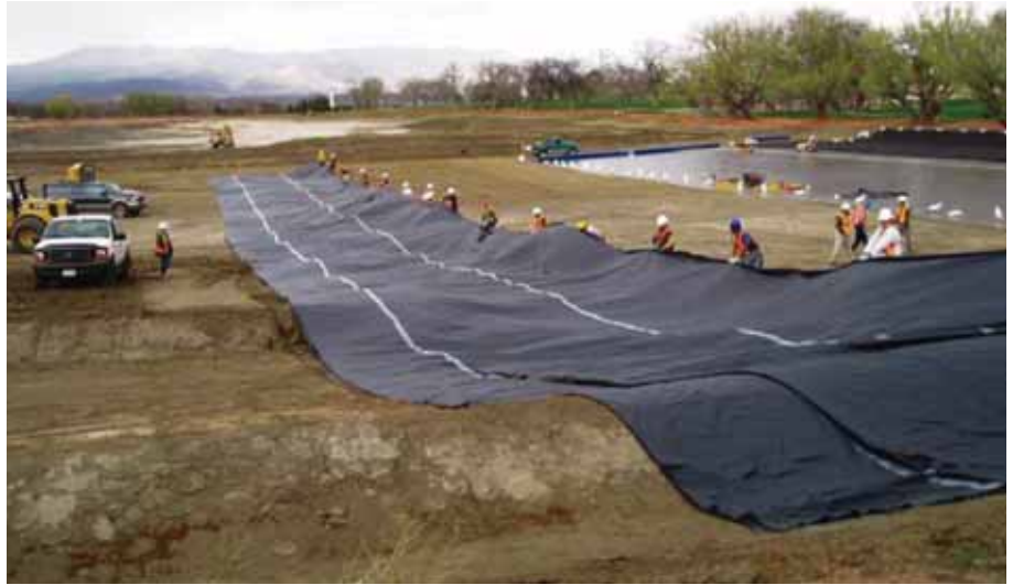
Photo 4 | The large PVC panels were unfolded and deployed.
