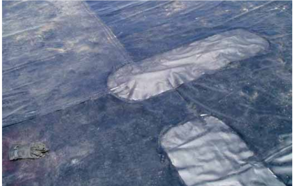
Photo 6 | Two examples of patches for destructive samples.
