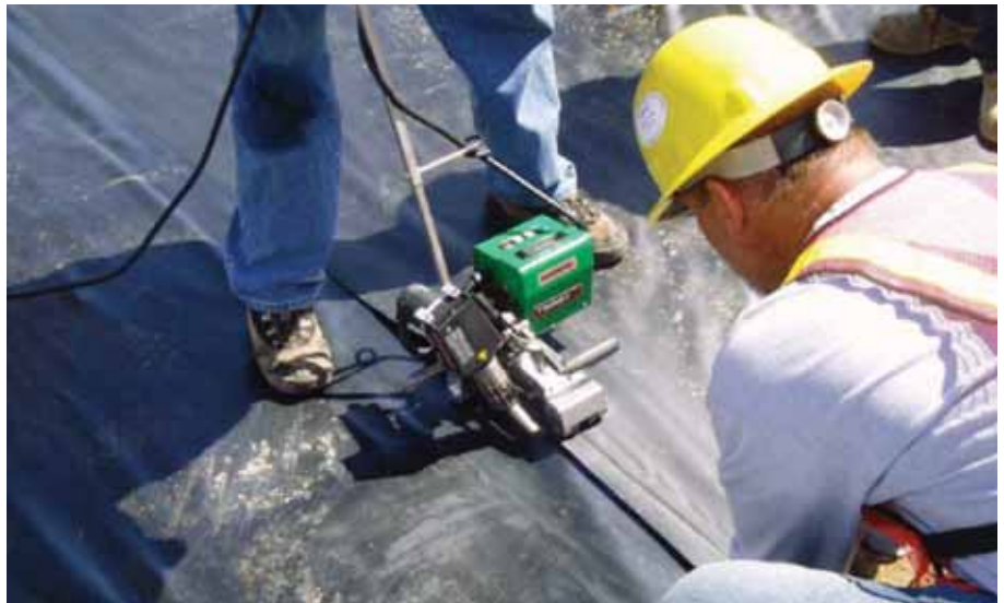
Photo 5 | Air-channel testing has been gaining popularity and has advantages over destructive testing.
