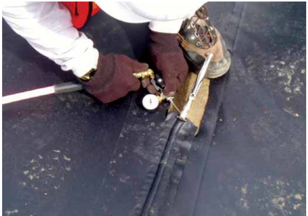
Photo 7 | An inflated field seam with no defects in the welds.
