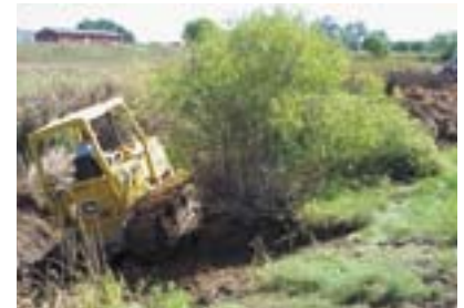
Photo 1: Willow tree and cattails being removed for geomembrane exhumation.
