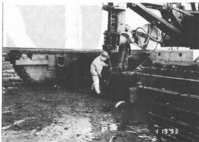
Fig. 5 Vertical Strip Drain Equipment at Craney Island
