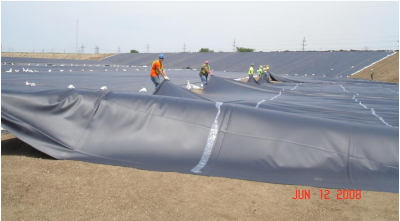
Figure 3 – Fabricated geomembrane panels being unfolded and deployed
