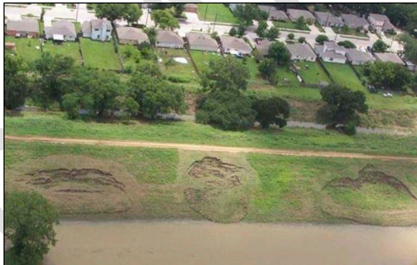
Figure 10. Photograph of shallow slides in levee system embankment
