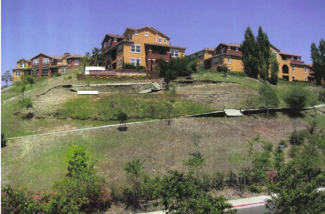
Figure 4. Slide in compacted fill slope after six years.
