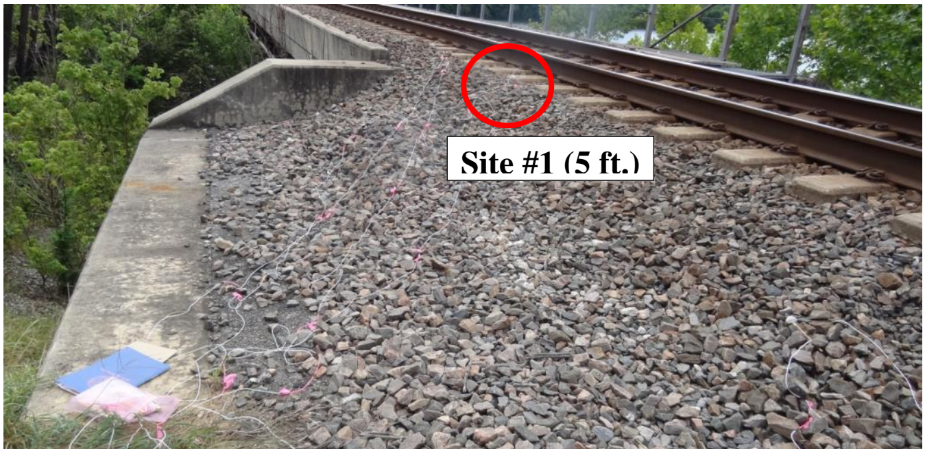
Figure 4: Photograph of the east end bridge transition zone at Site #1.
