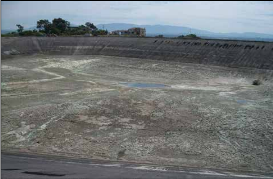
Figure 1. Reservoir drained immediately prior to starting construction.
