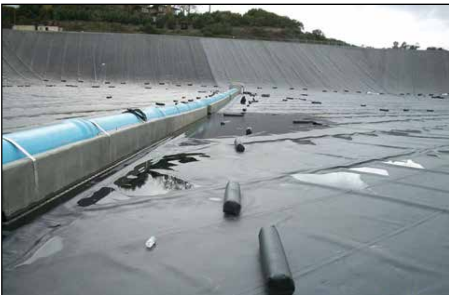
Figure 2. Geomembrane liner and inlet pipe extension during construction.
