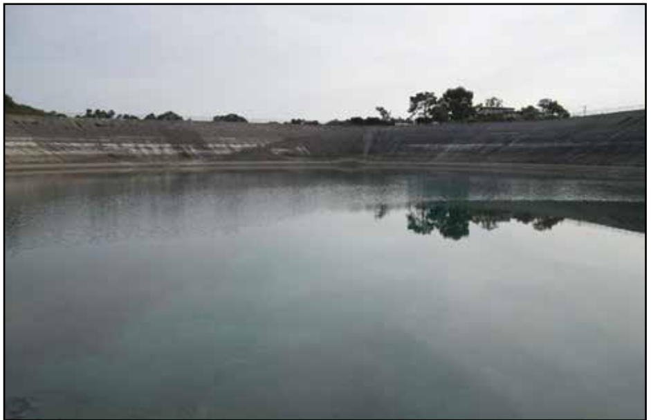
Reservoir in service draining prior to project.
